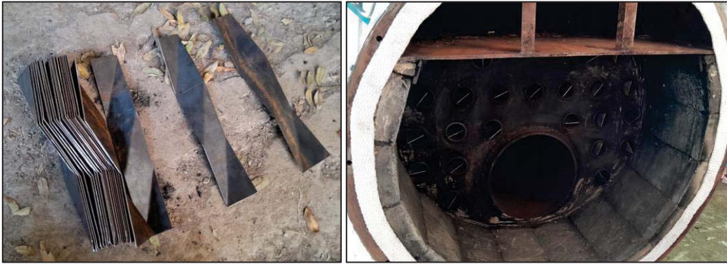
Fig. 3. Turbulator geometry and installation.
