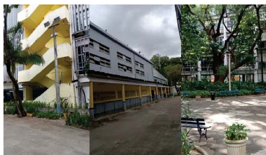
Fig.8. Outdoor Lighting Example. Source: CEFET, 2024.
